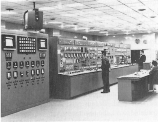
Figure 24.23 Control room of the 540 MW generator set. (Courtesy of General Electric)
